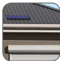
Roof Mounted Unit
